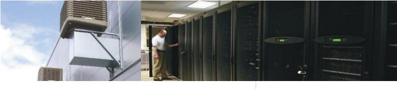
Workspace Technology's Modular Data Centre solution was delivered to the University 'server ready' - pre-engineered and wired ready for instant deployment of servers. As the MDC is self-contained it arrived on-site complete with cabinets, cooling, UPS and power distribution completely built based upon Workspace Technology's EcoDesignTM strategy designed to reduce carbon emissions through design and technology.
